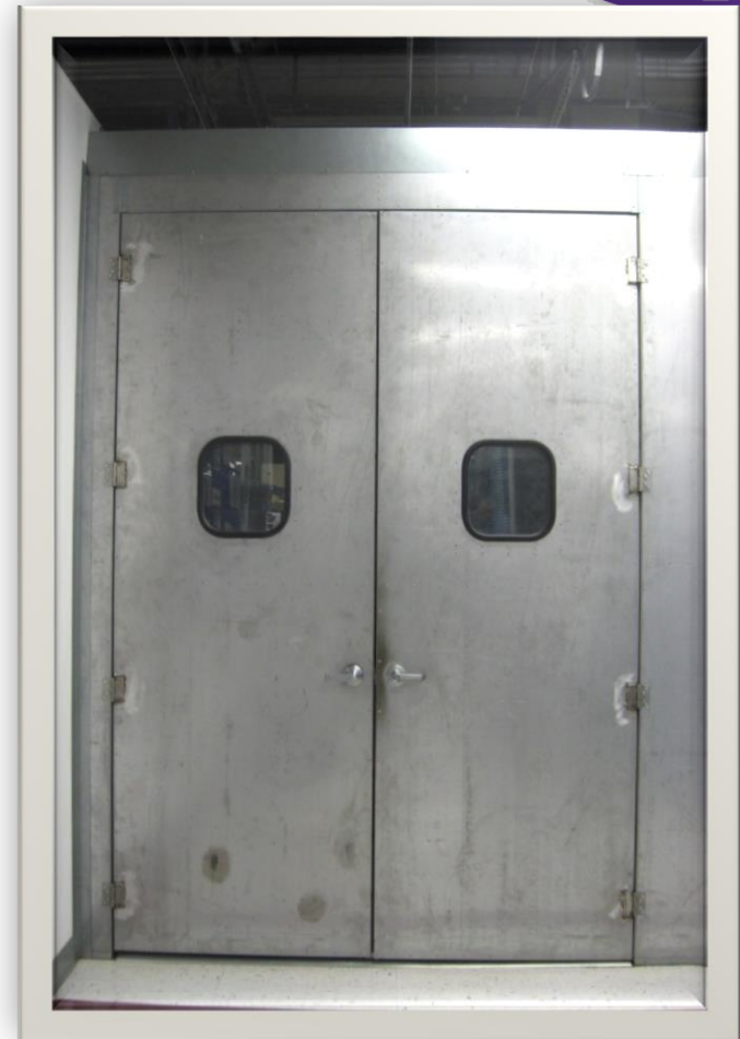
Control Room Enclosed
